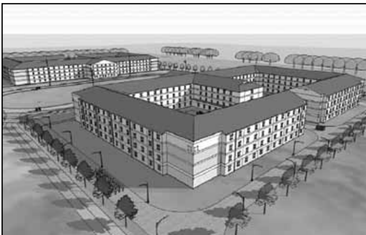
The Medical Education Training Complex at Fort Sam Houston in San Antonio, TX is a LEED certified project that meets the Army's stringent requirements for sustainability and low air infiltration, resulting in better indoor air quality and exceptional energy efficiency. Totalling over one million sq. ft., it is the largest modular project in North America and one of the biggest in the world. Photo courtesy Warrior Group.
