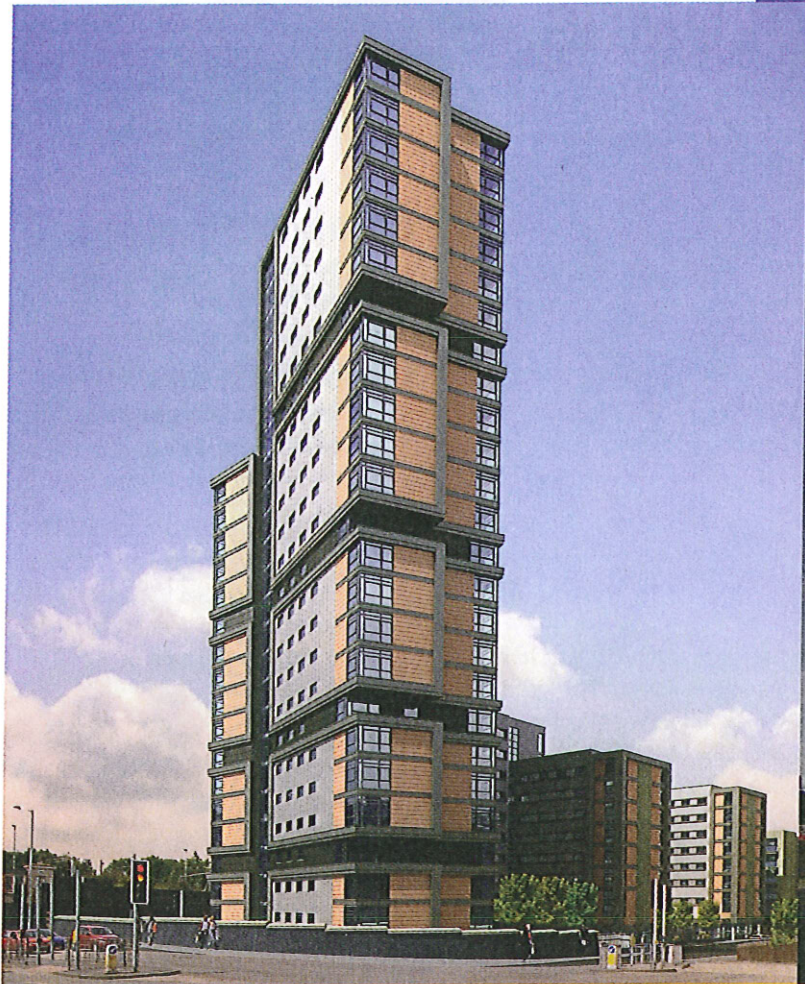
Located in Wolverhampton, UK, this modular student housing project, built in 27 weeks, would have taken 24 months using traditional site-built methods.
